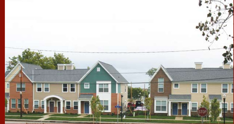
Tremont Pointe Phase I construction consists of 102 mixed-income garden and townhouse rental units.
